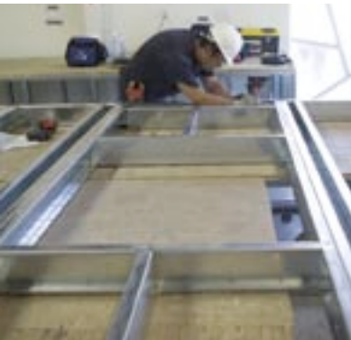
PLANT, SITE PHOTOS: Steven Miller for Ecolite Concrete USA
